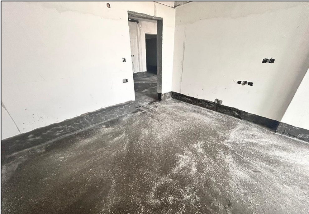
A 0905 – Water Proofing works in progress
