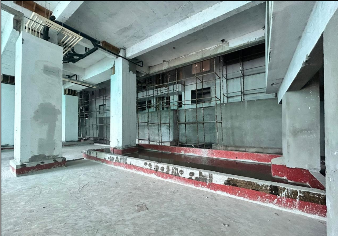
Arrival Area – Waterproofing works in progress
