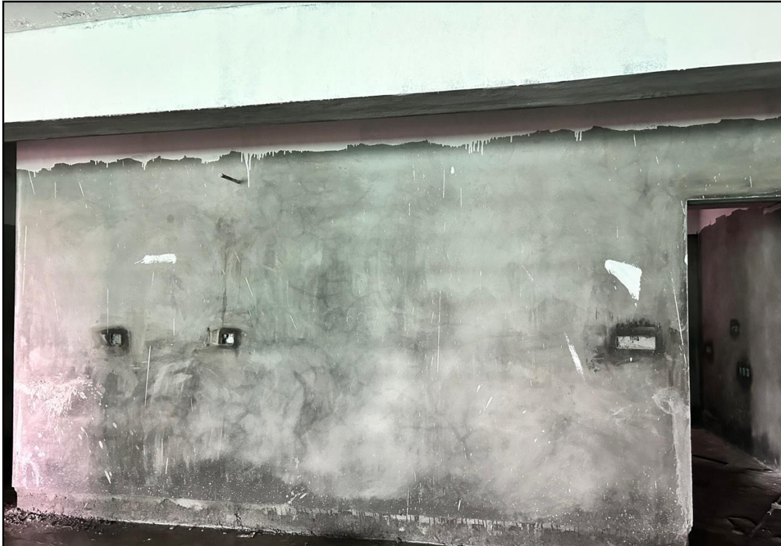
A 0710 – Internal Plastering works in progress
