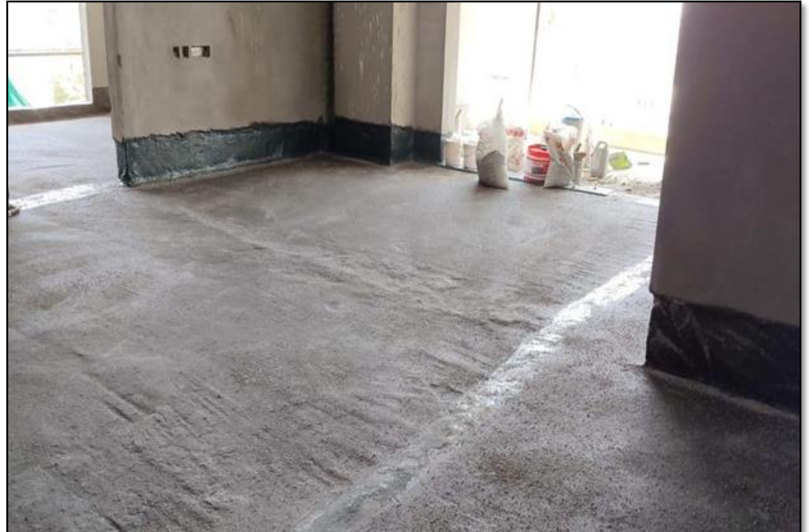
A 0804 – Waterproofing works in progress
