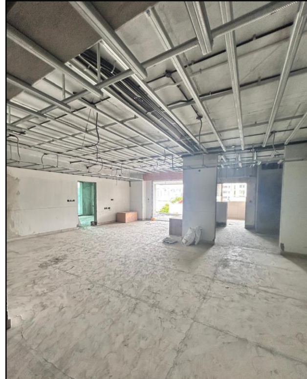
A 0404 – False Ceiling works in Progress
