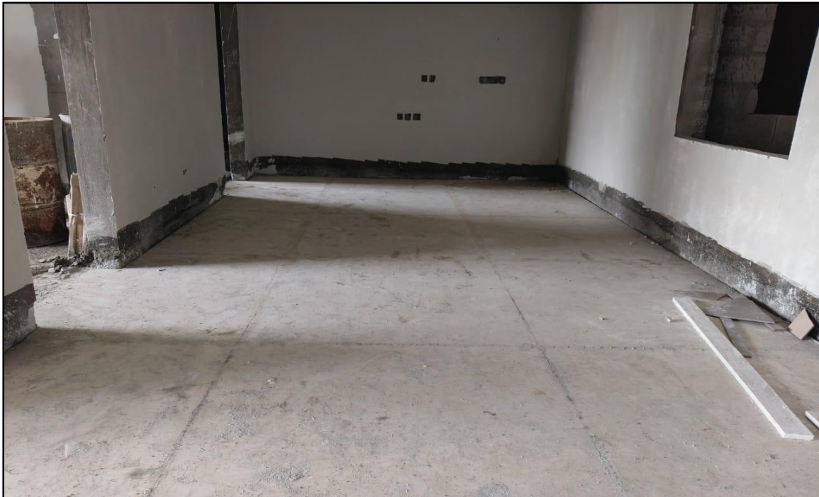
A 0505 – Flooring works in Progress
