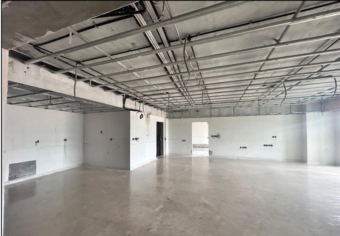
A 0403 – False Ceiling works in Progress
