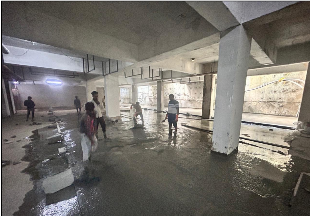
Basement – Flooring works in progress
