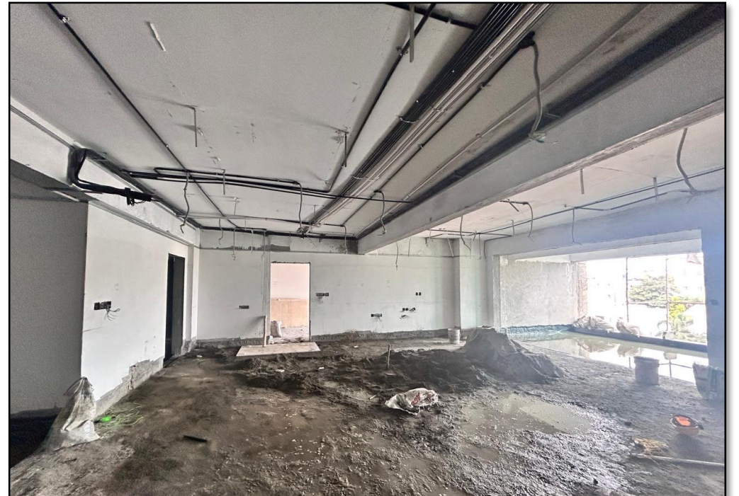
A 0503 – Flooring works in Progress
