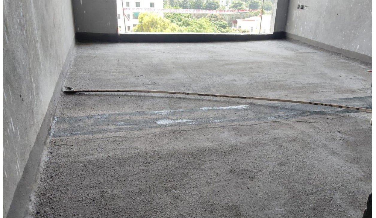
A 0806 – Waterproofing works in Progress
