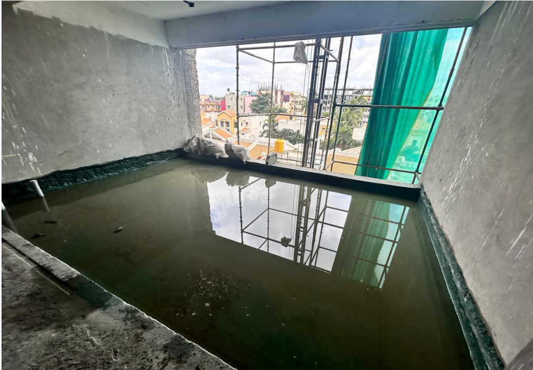
A 0508 – Waterproofing works in Progress
