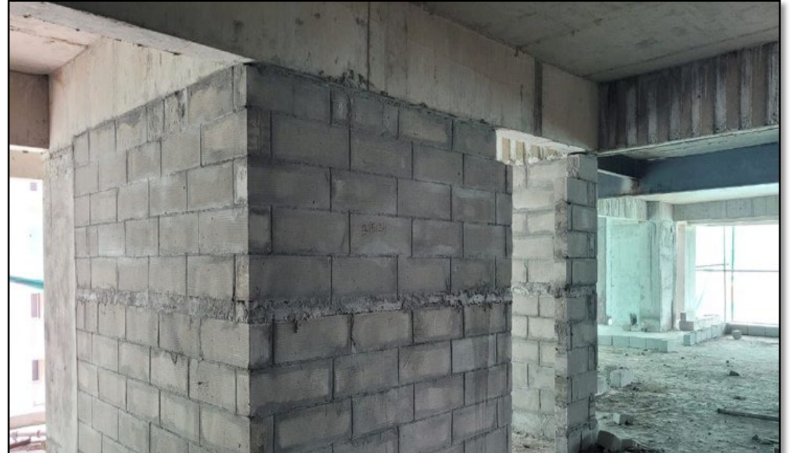
A 1204 – Block works in Progress
