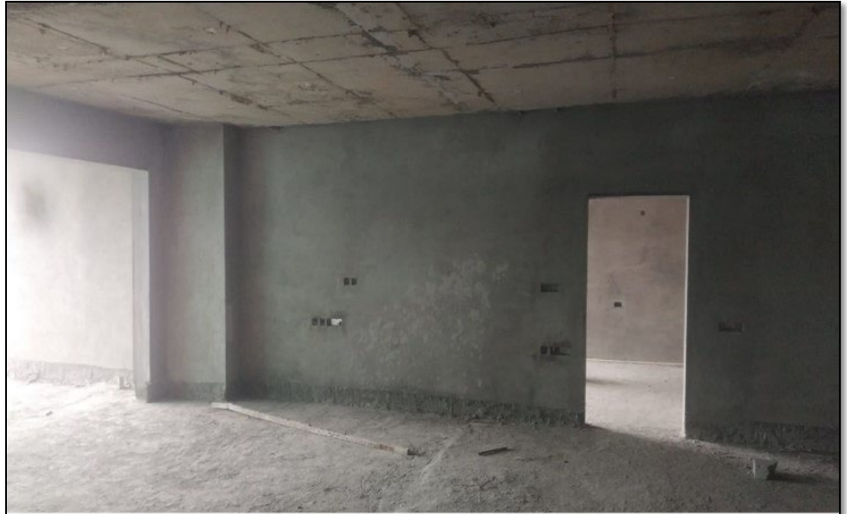
A 0506 – Plastering works in Progress
