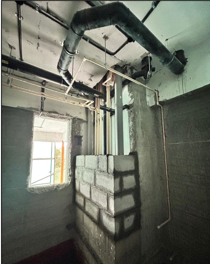
A 0201 – PHE works in Progress
