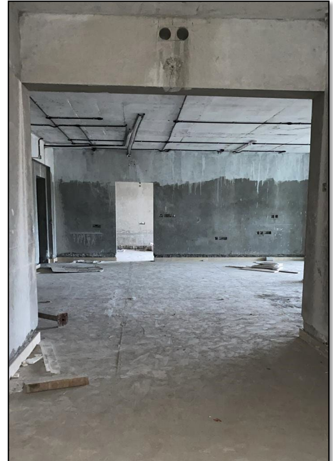
A 0403 – Marble Works in Progress
