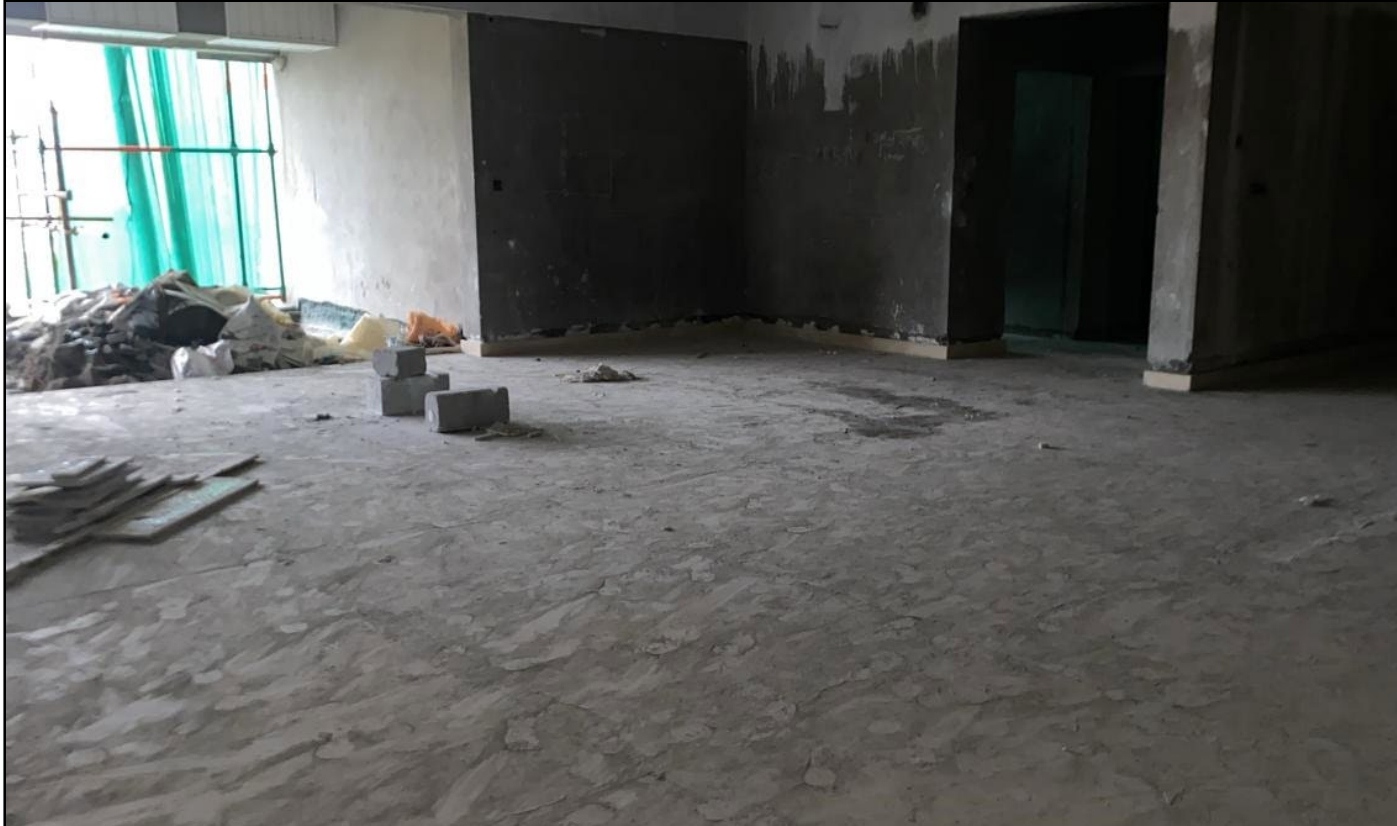
A 0403 – Marble Works in Progress
