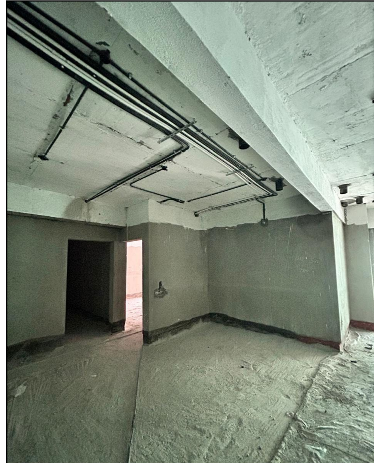
A 0204 – Ceiling conduiting works in Progress
