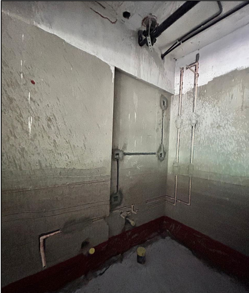
A 0404 – Block works in Progress
