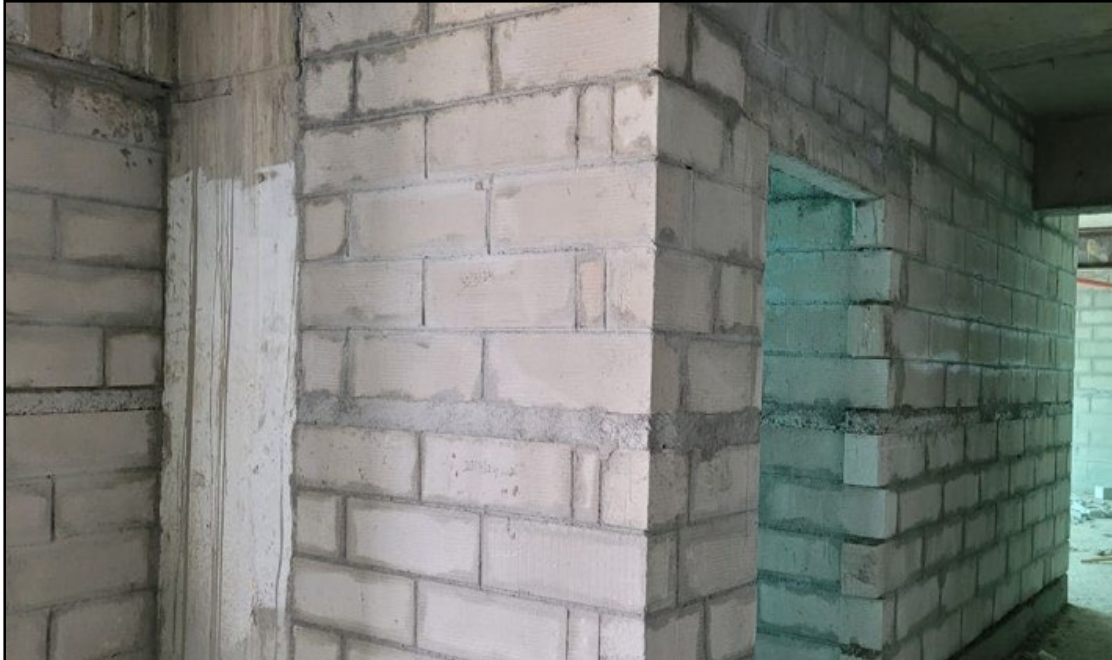
A 1010 – Block works in Progress
