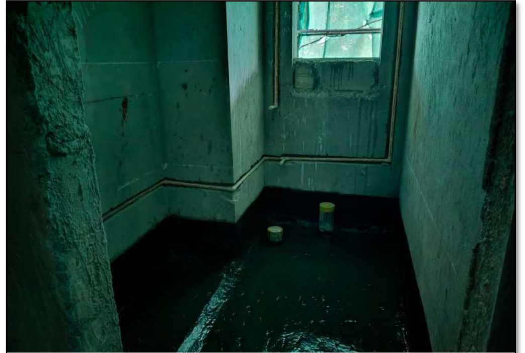
A 0206 – Water Proofing works in Progress
