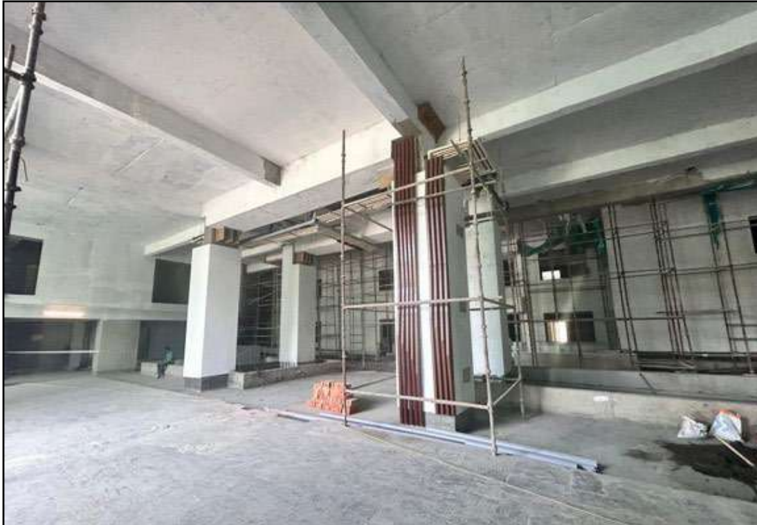
Entrance Lobby – Cladding works in progress
