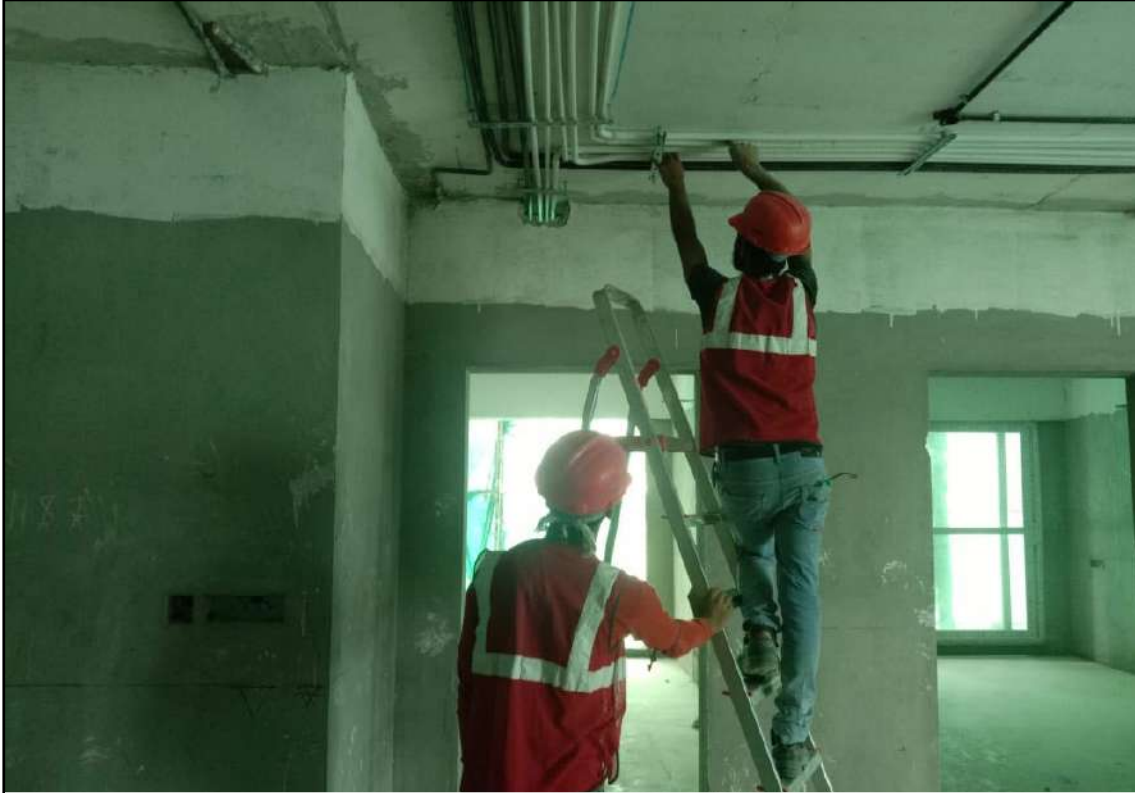
A 0301 – Electrical works in Progress
