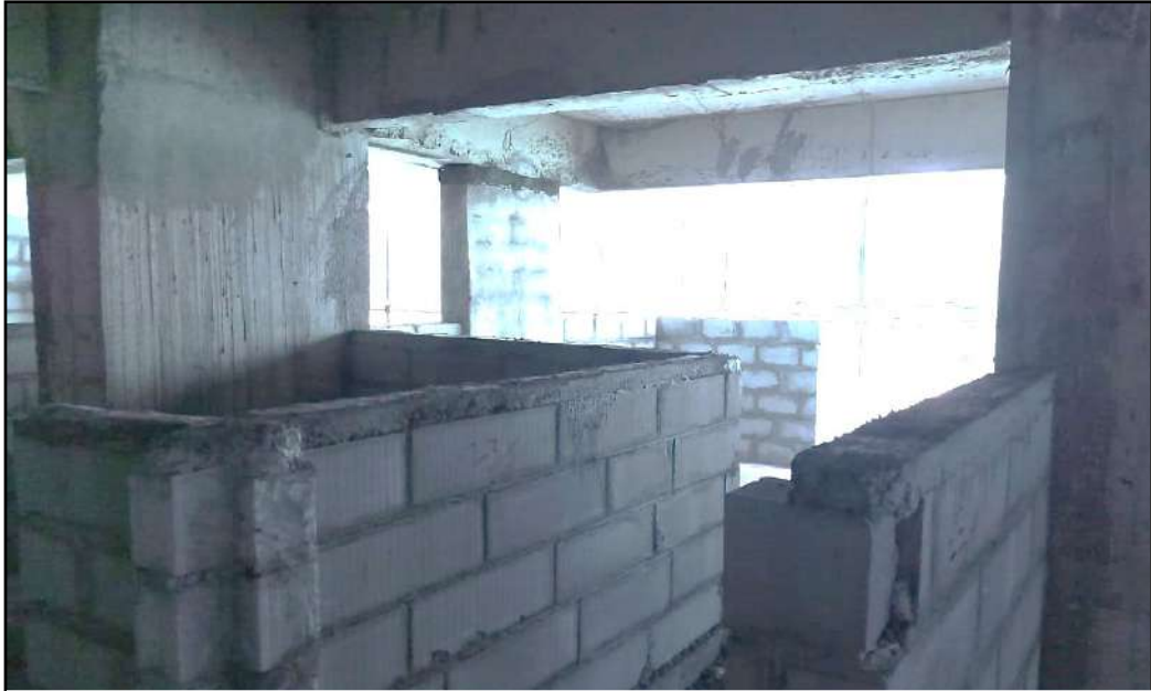
A 1010 – Block works in Progress
