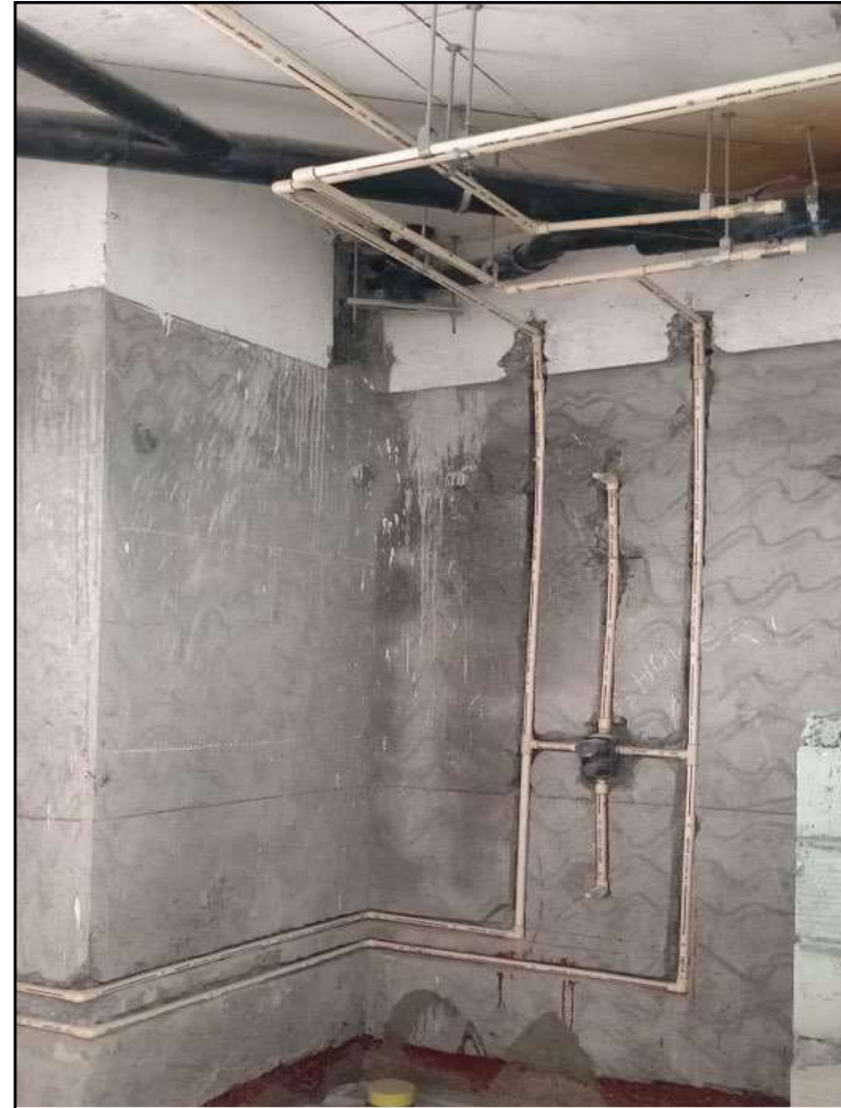
Level 4 – PHE works in Progress
