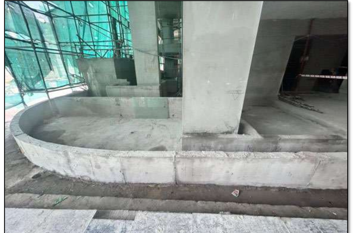
Entrance Lobby – Water proofing works in progress
