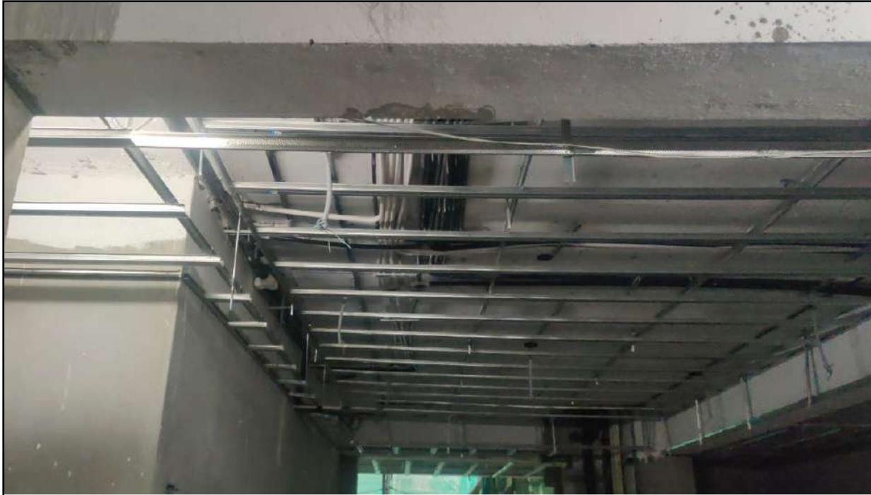
A 0209 – False Ceiling works in Progress
