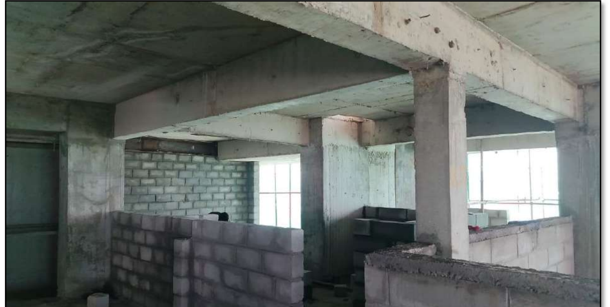
A 1204 – Block works in Progress
