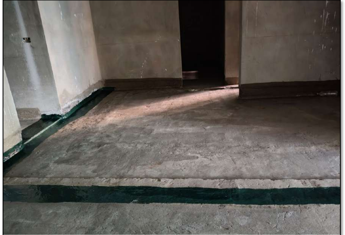
A 0209 – Water Proofing works in Progress
