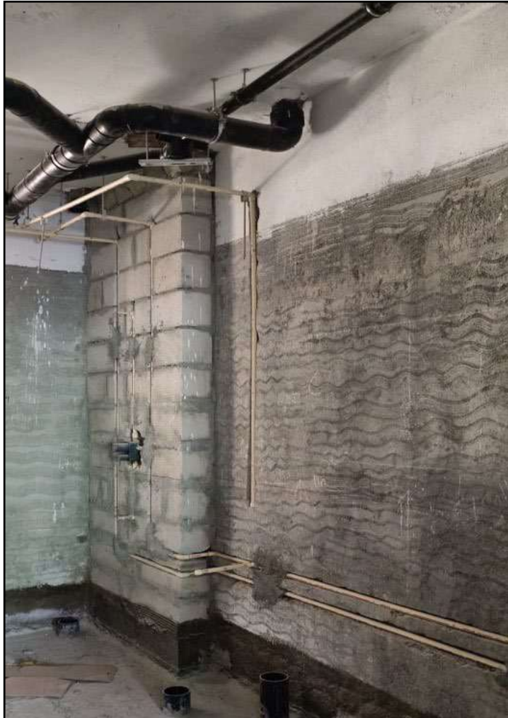
Level 3 – PHE works in Progress
