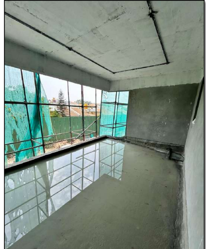
A 0301 - Waterproofing Works in Progress
