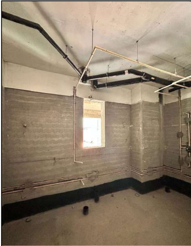
PHE Works in Progress
