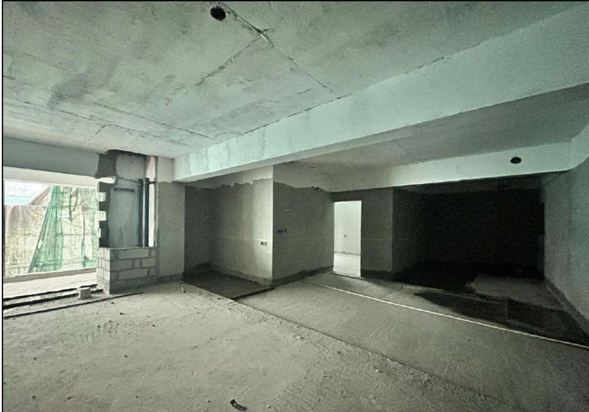
A 0404 - Waterproofing Works in Progress
