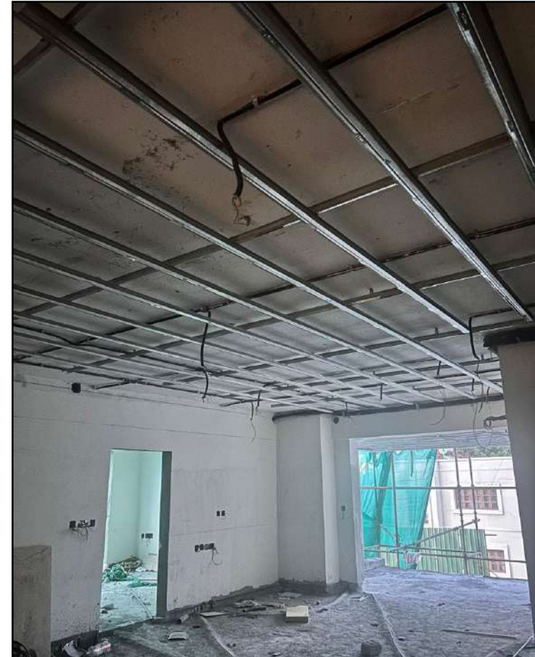
A 0304 – False Ceiling Works in Progress
