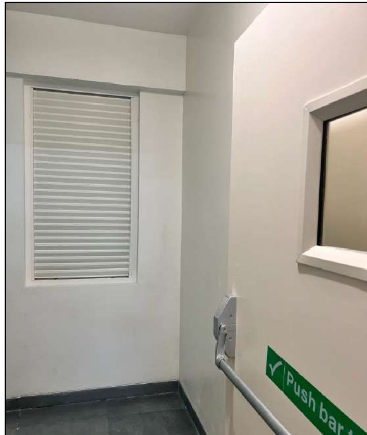
Common Area Staircase Fire Door Installed
