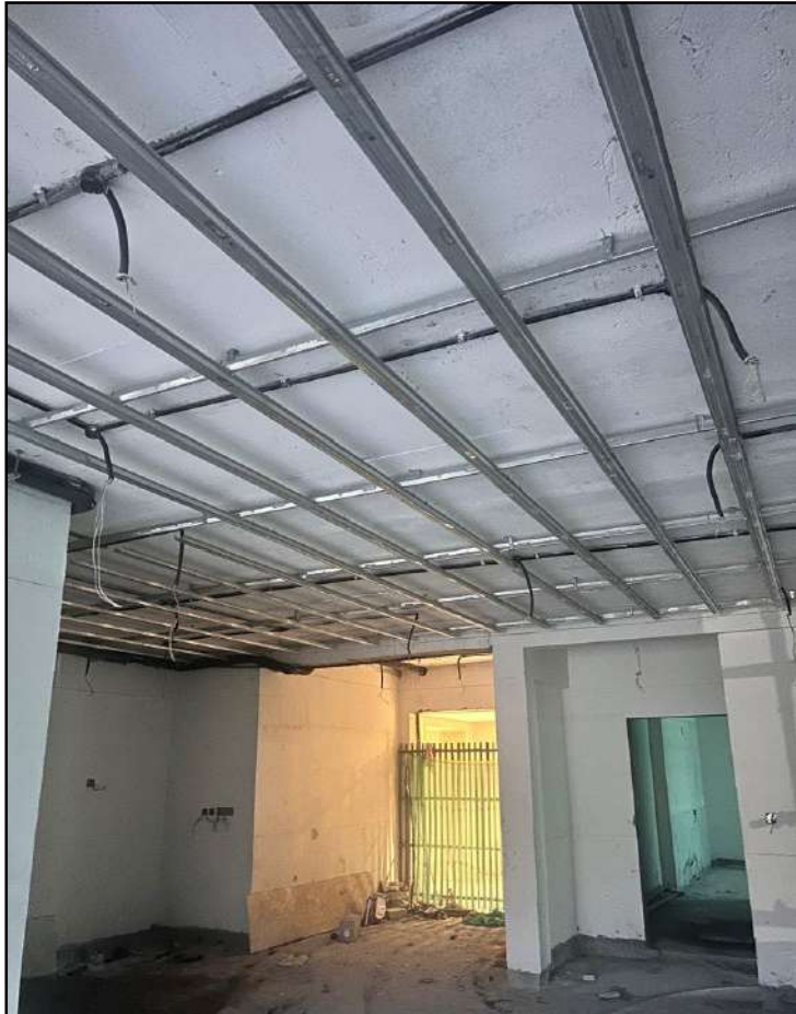
A 0304 – False Ceiling Works in Progress
