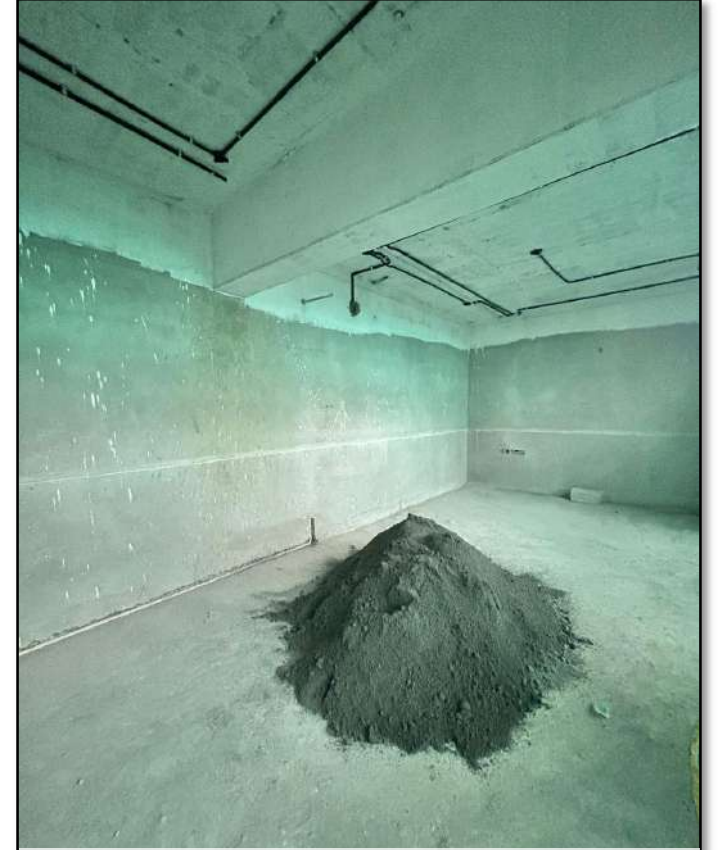
A 0109 – Marble Flooring Works in Progress
