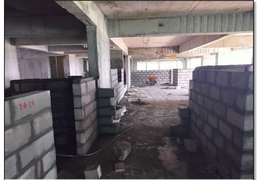
A 0901 - Block Masonry Works in Progress
