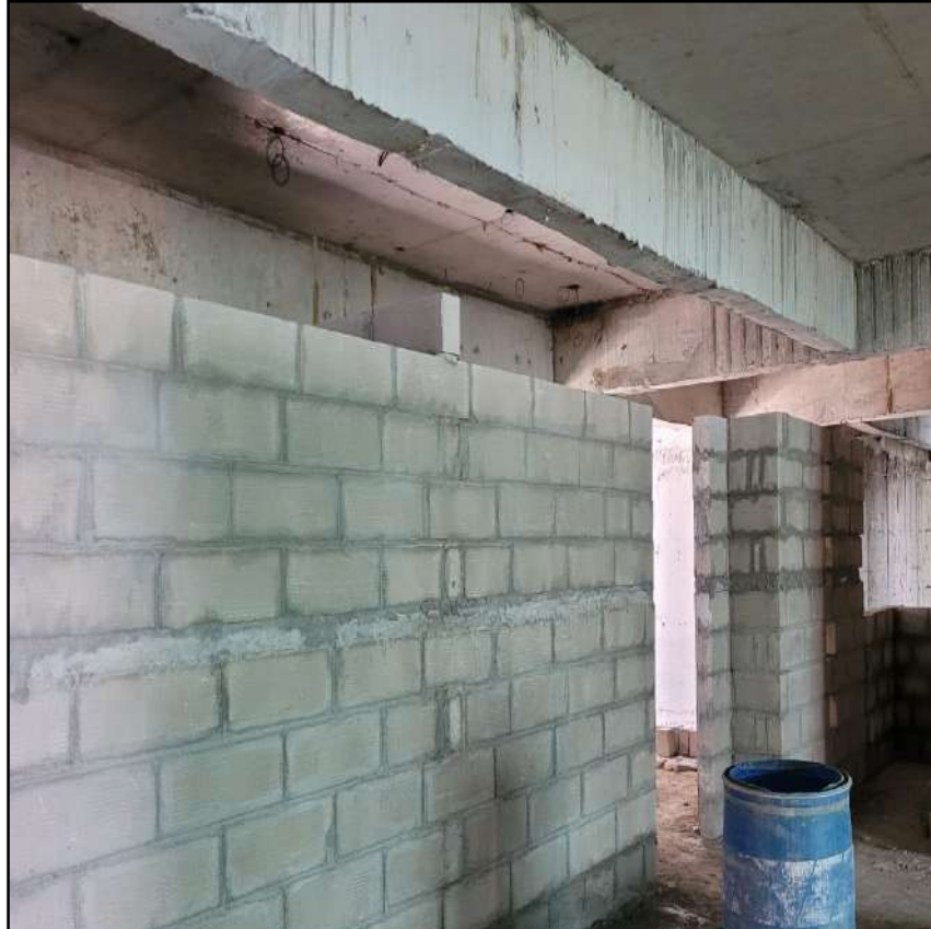
A 0605 - Block Masonry Works in Progress
