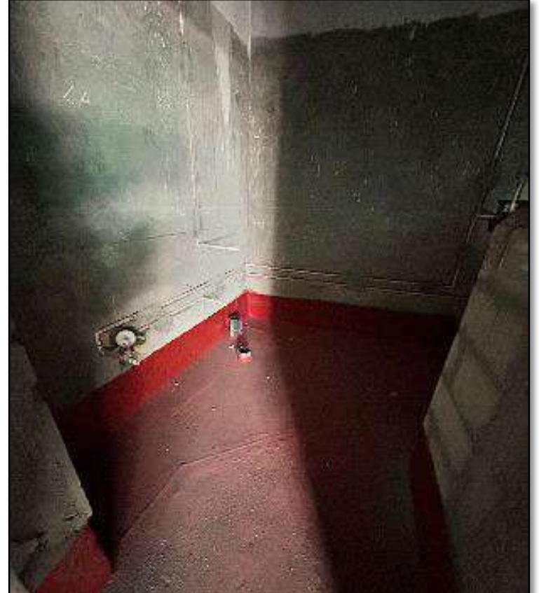
A 0109 - Waterproofing Works in Progress
