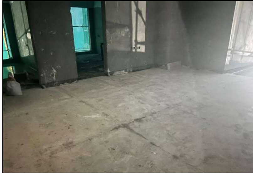
A 0301 – Marble Flooring Works in Progress
