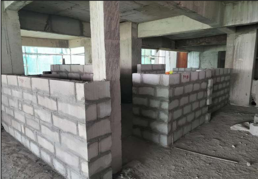
A 1102 - Block Masonry Works in Progress
