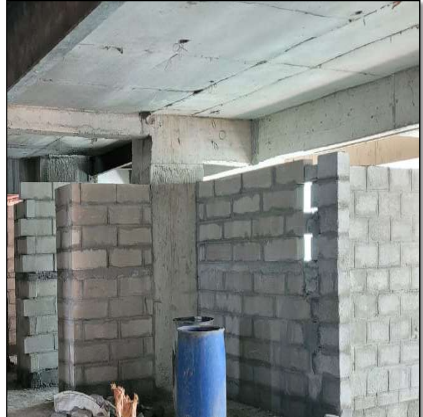
A 0803 - Block Masonry Works in Progress
