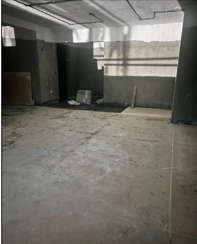
A 0301 – Marble Flooring Works in Progress
