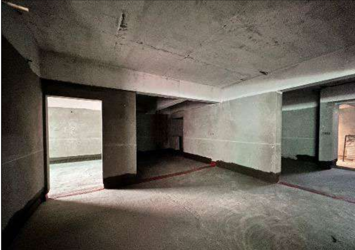
A 0106 - Waterproofing Works in Progress
