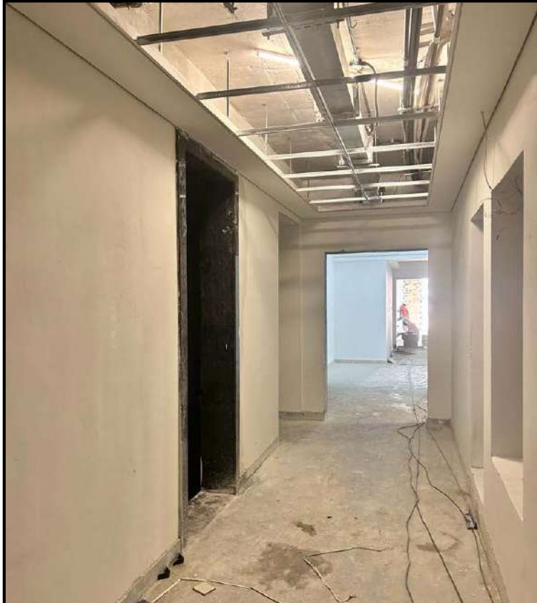
Common Area Service Lobby, False Ceiling works in progress
