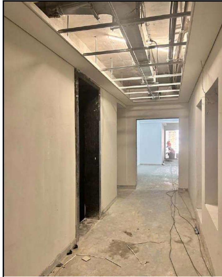
Common Area Service Corridor works in Progress
