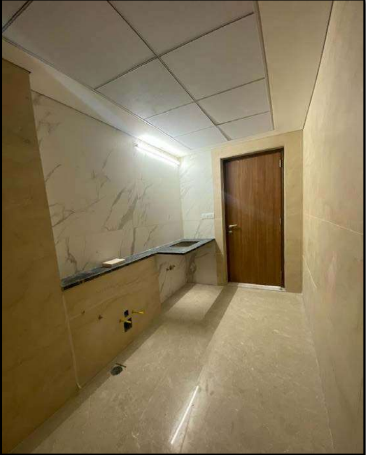
Toilet Finishing in Progress
