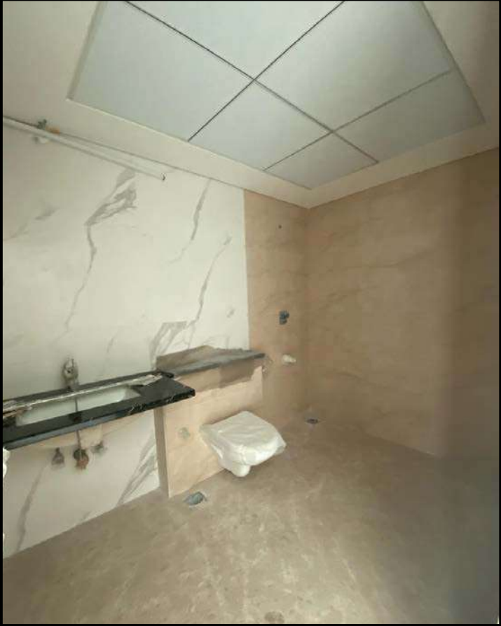
Toilet Finishing in Progress
