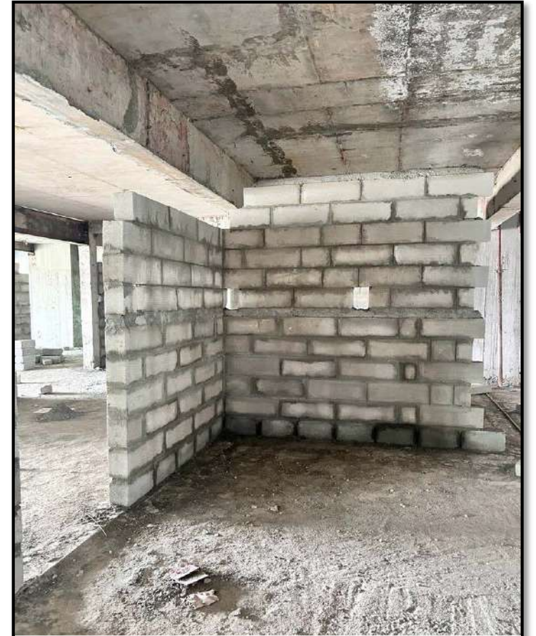
Level 8 th & 9 th Floor Civil works in Progress
