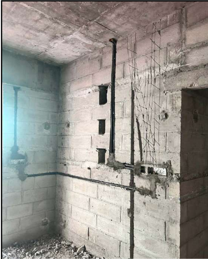
Electrical Works in Progress
