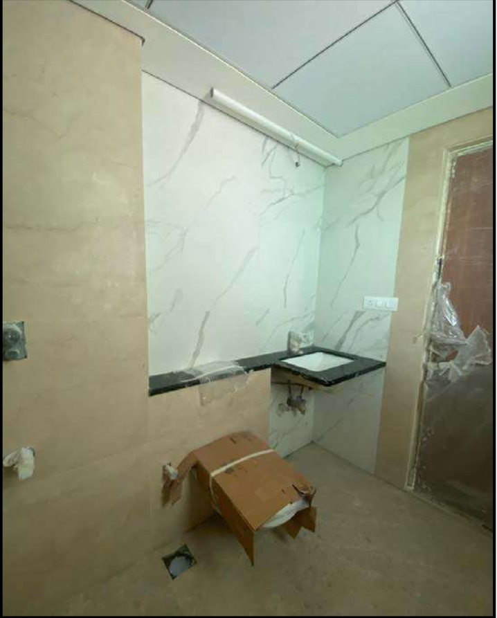
Toilet Finishing in Progress
