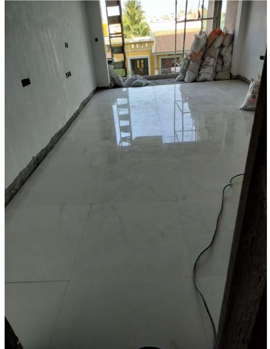
Base for Wooden Flooring works in progress
