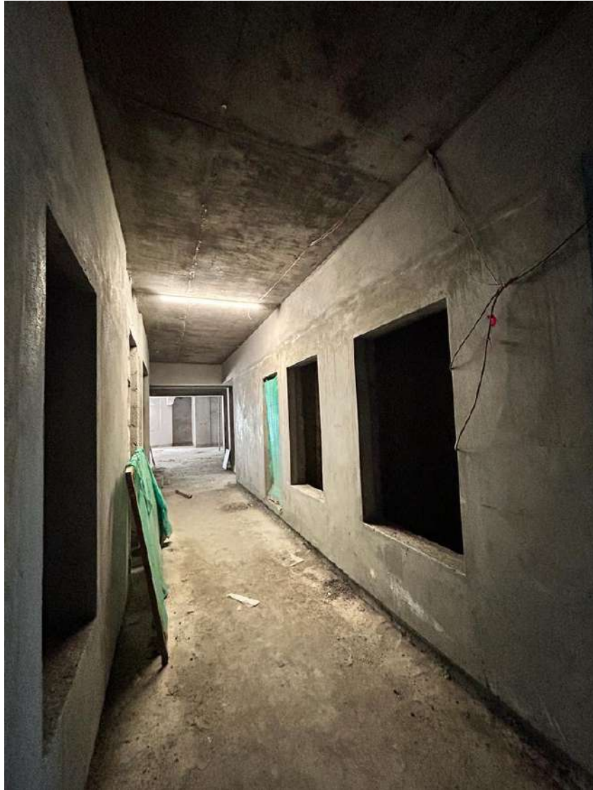
Lobby Plastering Works in Progress
