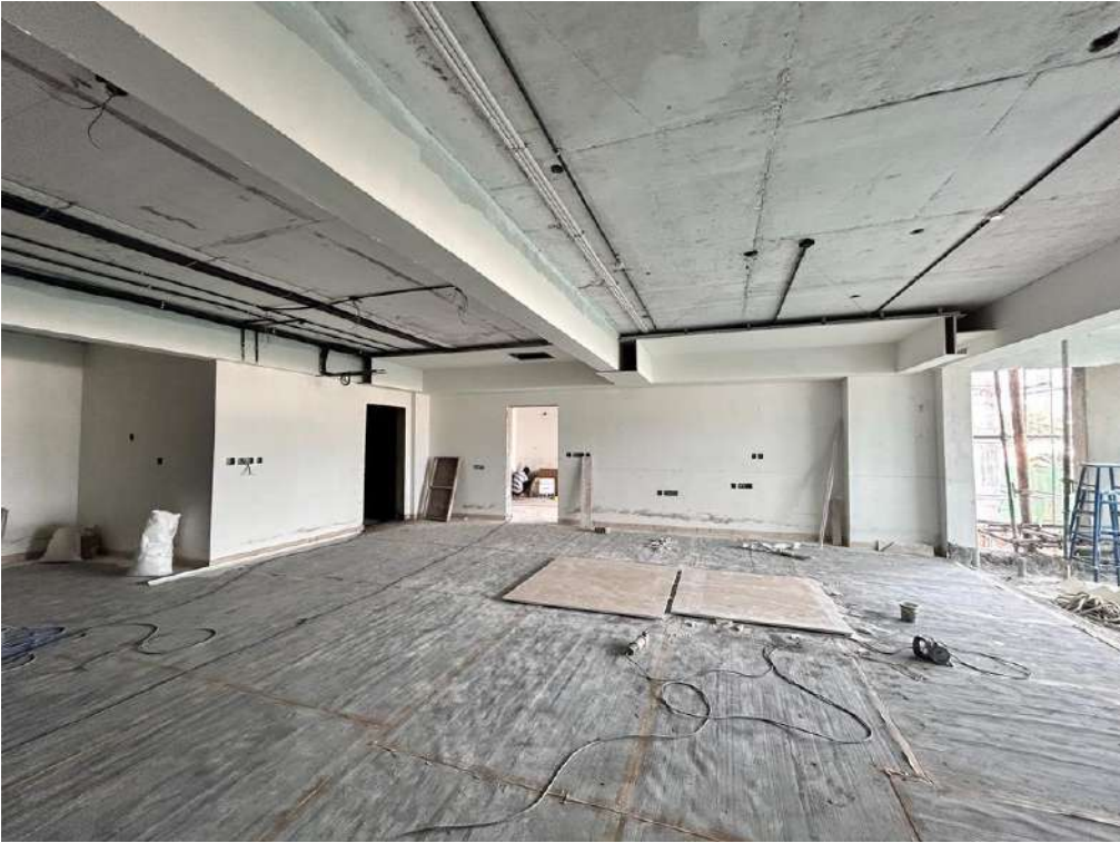
False Ceiling Works in Progress
