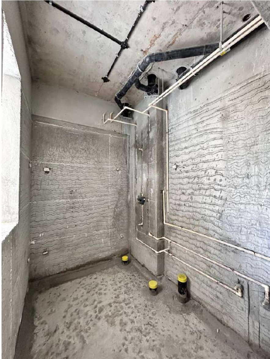
Toilet PHE works in Progress
