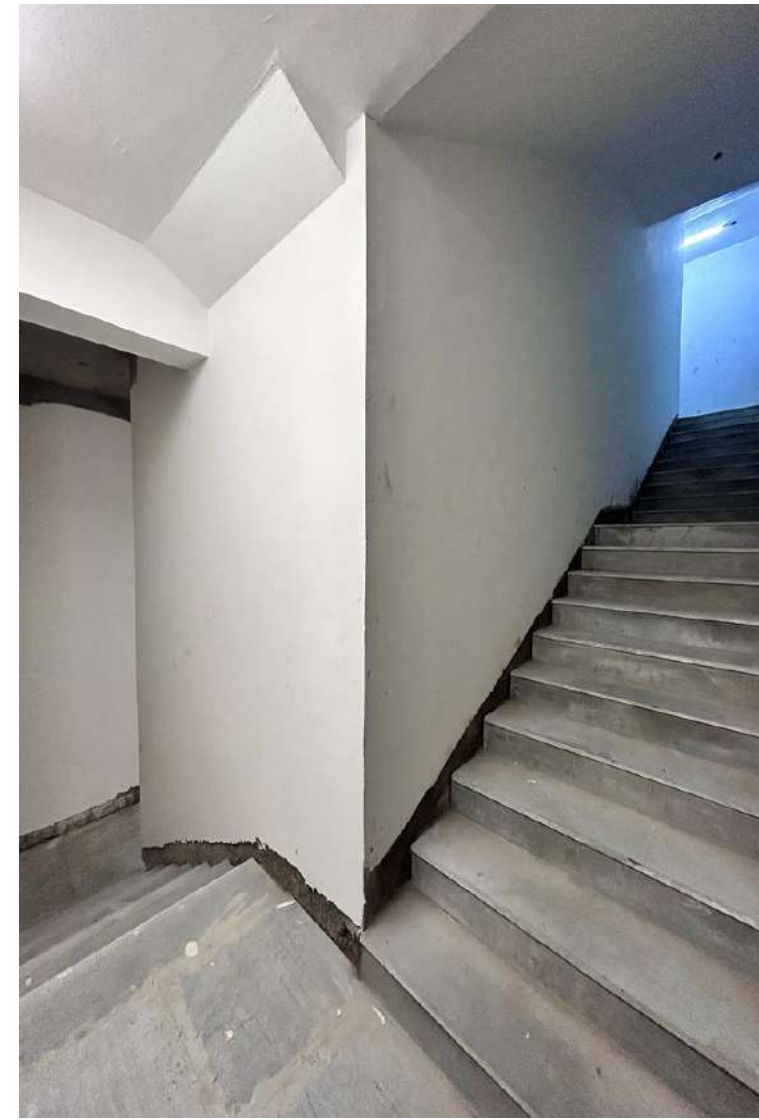
Staircase Flooring and Putty works in progress
