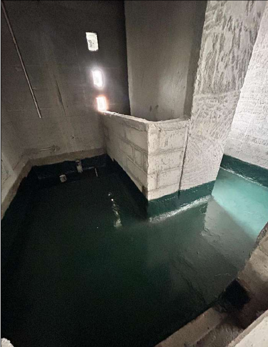
Toilet Waterproofing works in Progress
