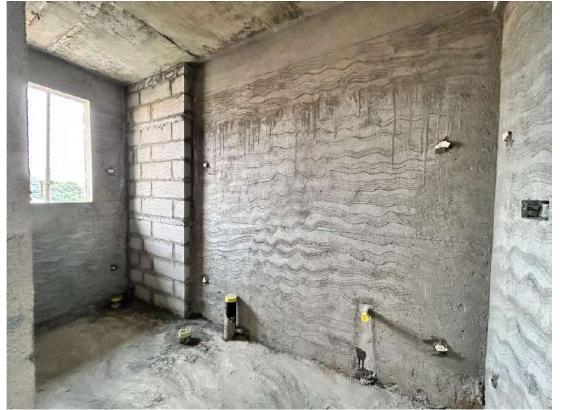
Toilet Plastering works in progress
