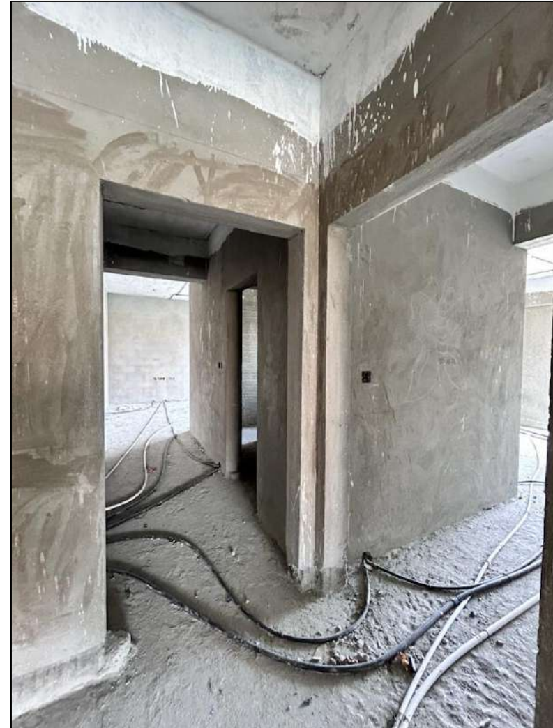
Unit Plastering works in progress
