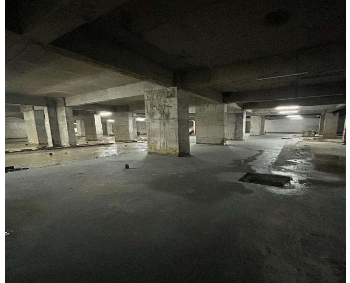
VDF Flooring and Primer works in Progress
